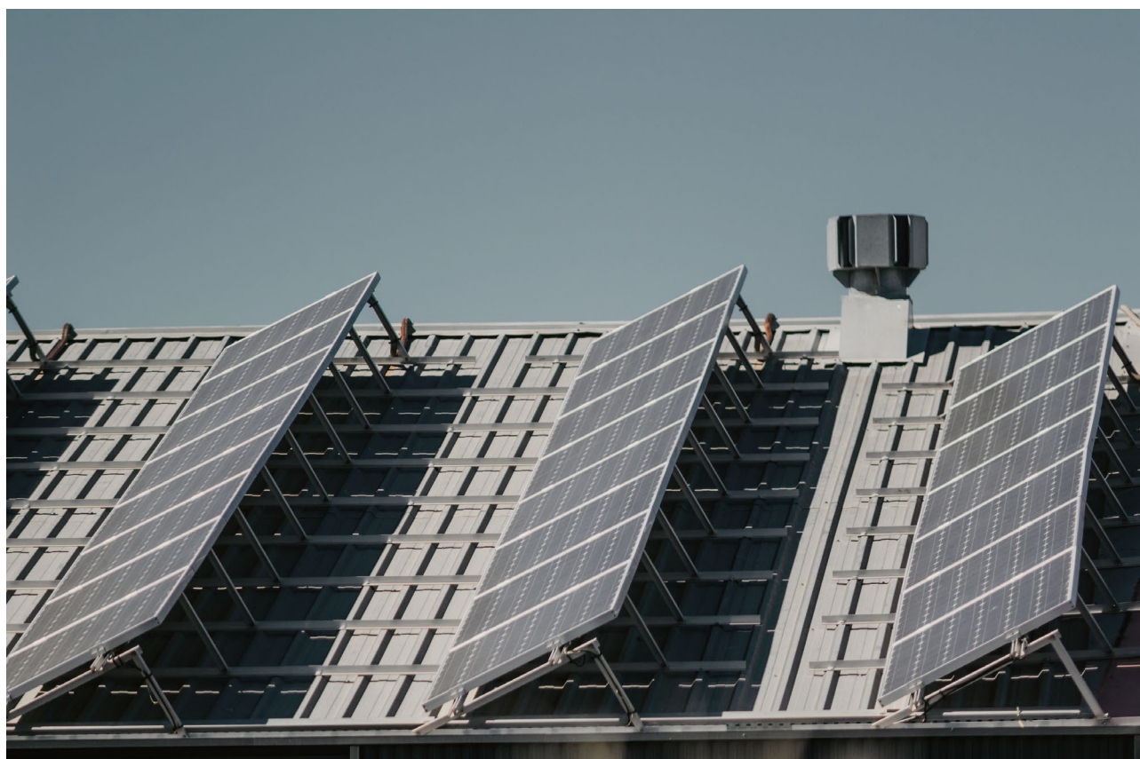
Installation of solar panels at Importaco's headquarters in Beniparrell.
